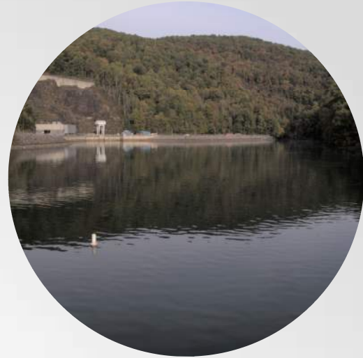
Bad Creek Pumped Storage Project USR Meeting | 101
