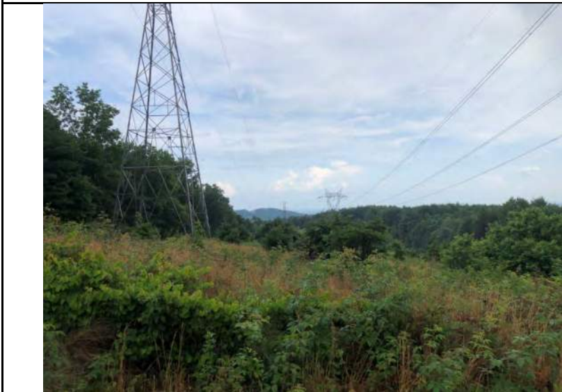
Photograph 27 – View of Study Area (Facing South)
