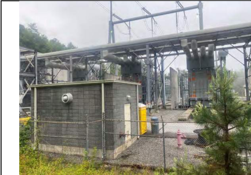
Photograph 1 – Bad Creek Hydro Station (Facing East)
