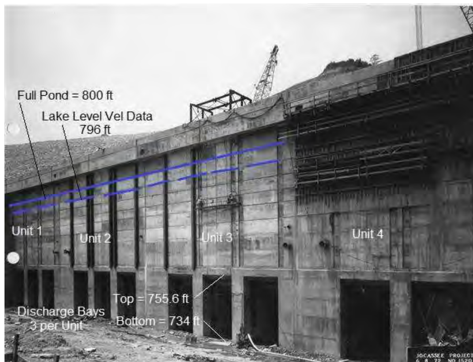
Figure 5. Construction photograph of JPSS discharge structure, with elevations.
