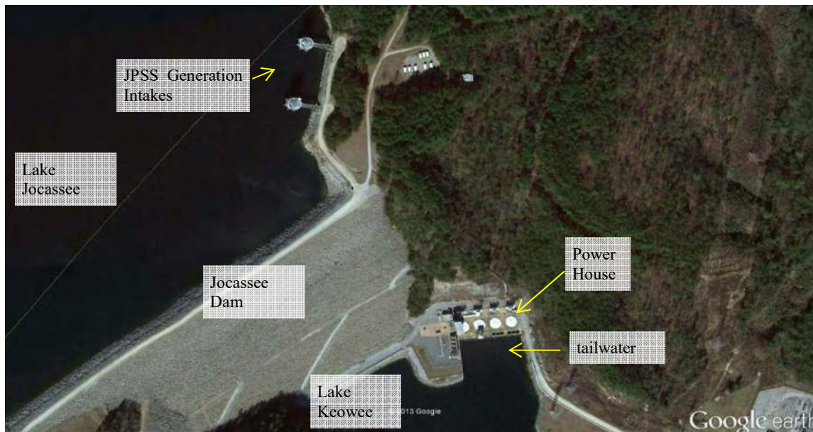
Figure 1. Aerial view of the Jocassee Pumped Storage Station.
