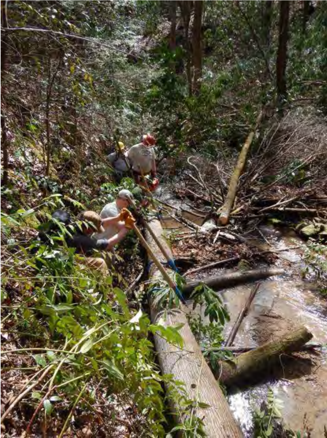
SCDNR brook trout habitat enhancement on Laurel Creek in progress
