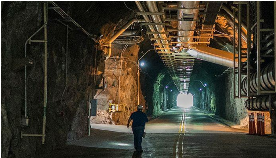
Figure 5.4-8. Bad Creek Entrance Tunnel (Source: Moore 2016)
