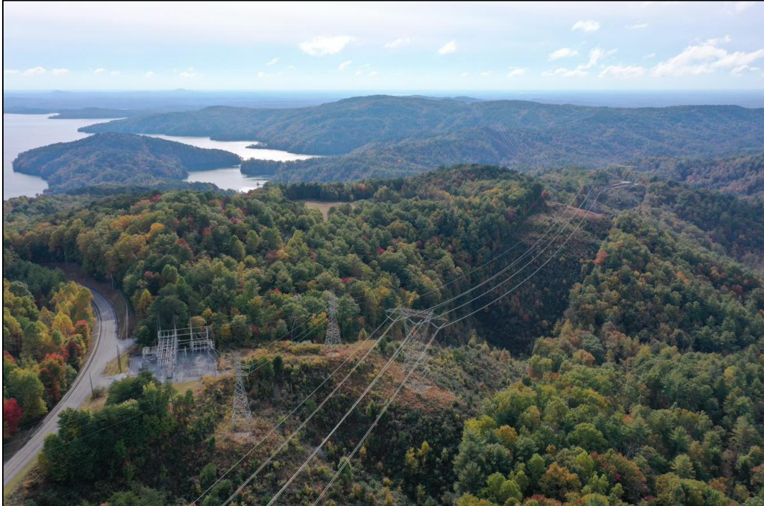
Figure 5.4-11. 525-kV Transmission Line and Corridor
