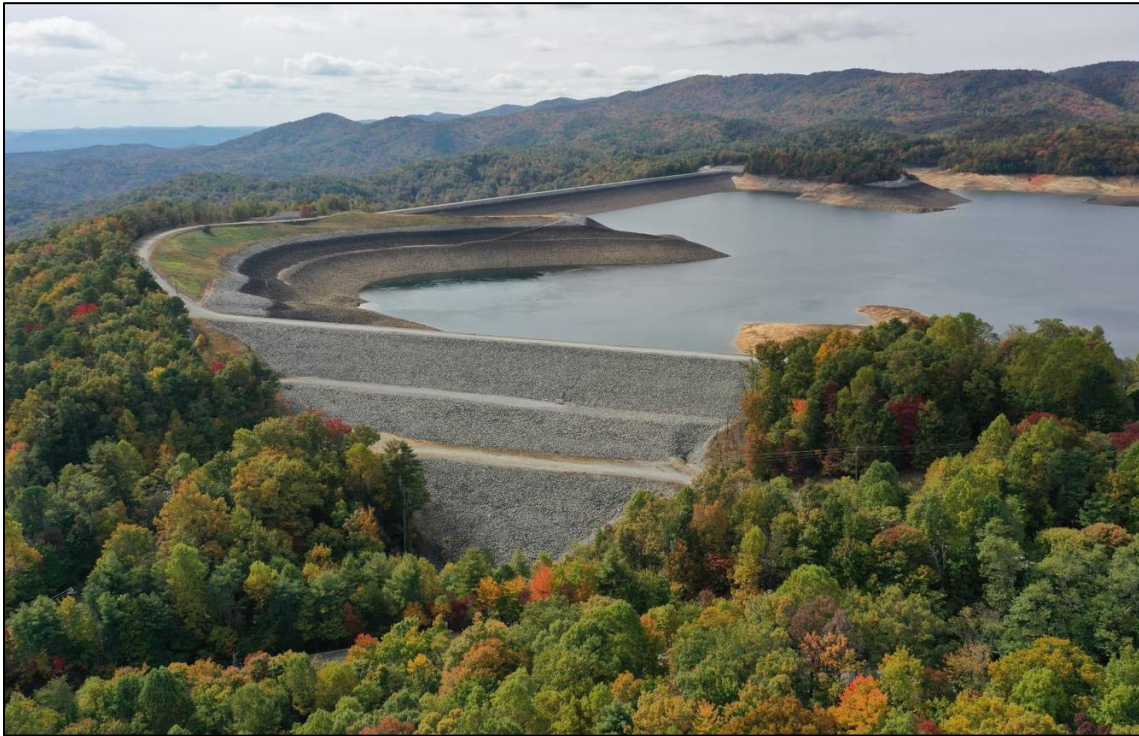
Figure 5.4-1. View of the Bad Creek Upper Reservoir
