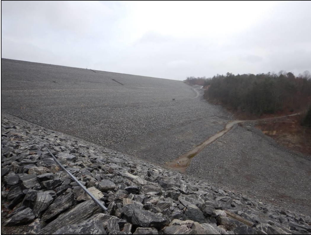
Figure 5.4-2. Downstream Face of Main Dam
