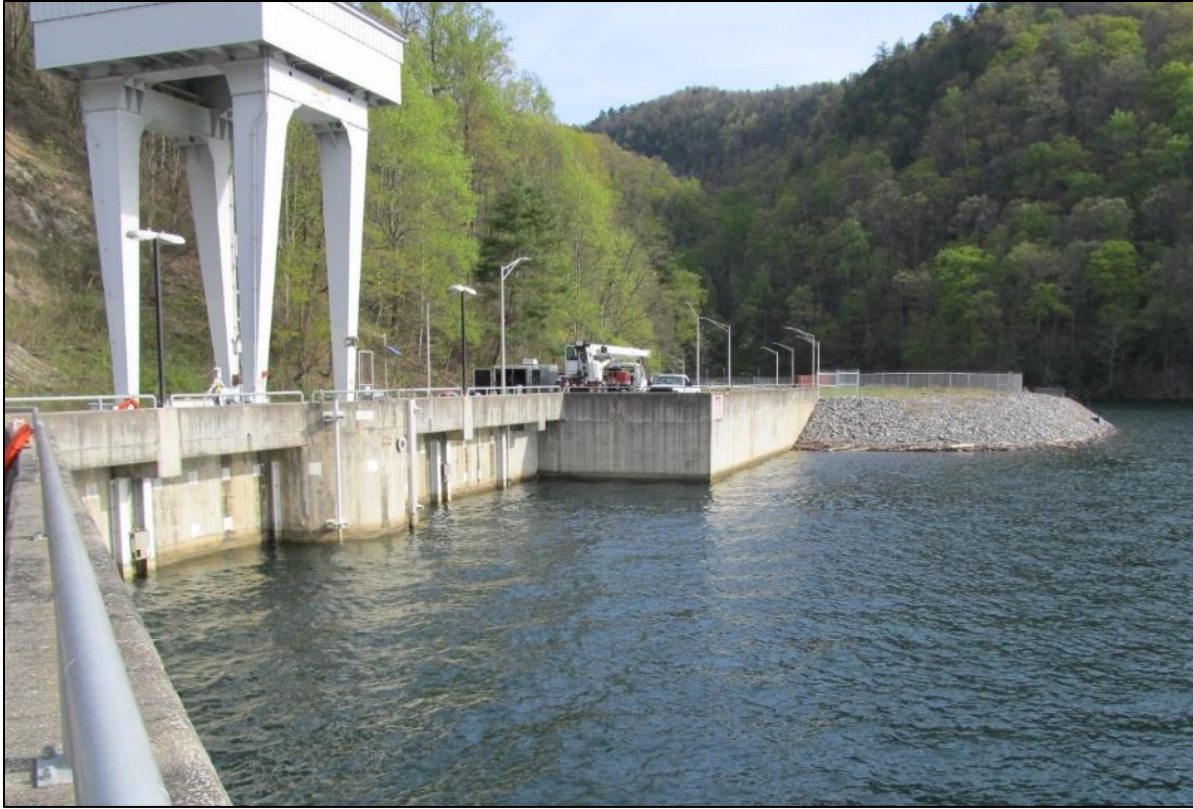
Figure 5.4-6. Lower Reservoir Inlet/Outlet Structure
