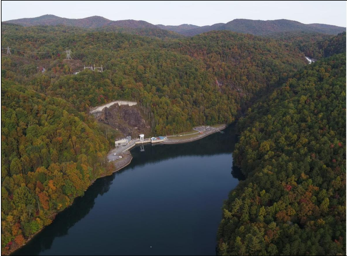
Figure 5.4-5. Lower Reservoir (Whitewater River Arm of Lake Jocassee), Inlet/Outlet Structure, and Powerhouse Portal Area
