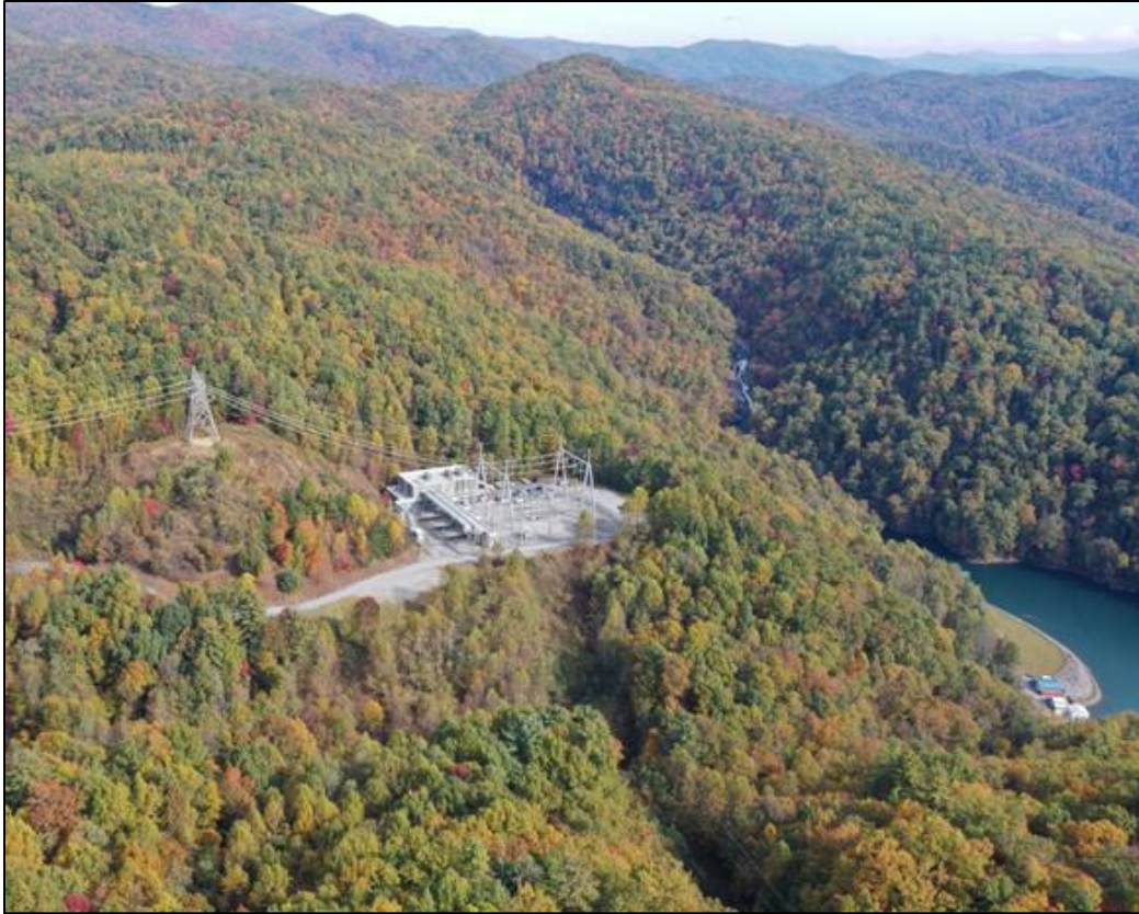
Figure 5.4-7. Aerial View of Bad Creek Switchyard
