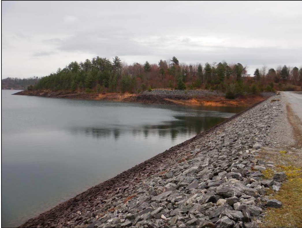
Figure 5.4-3. Upstream Face of the West Dam
