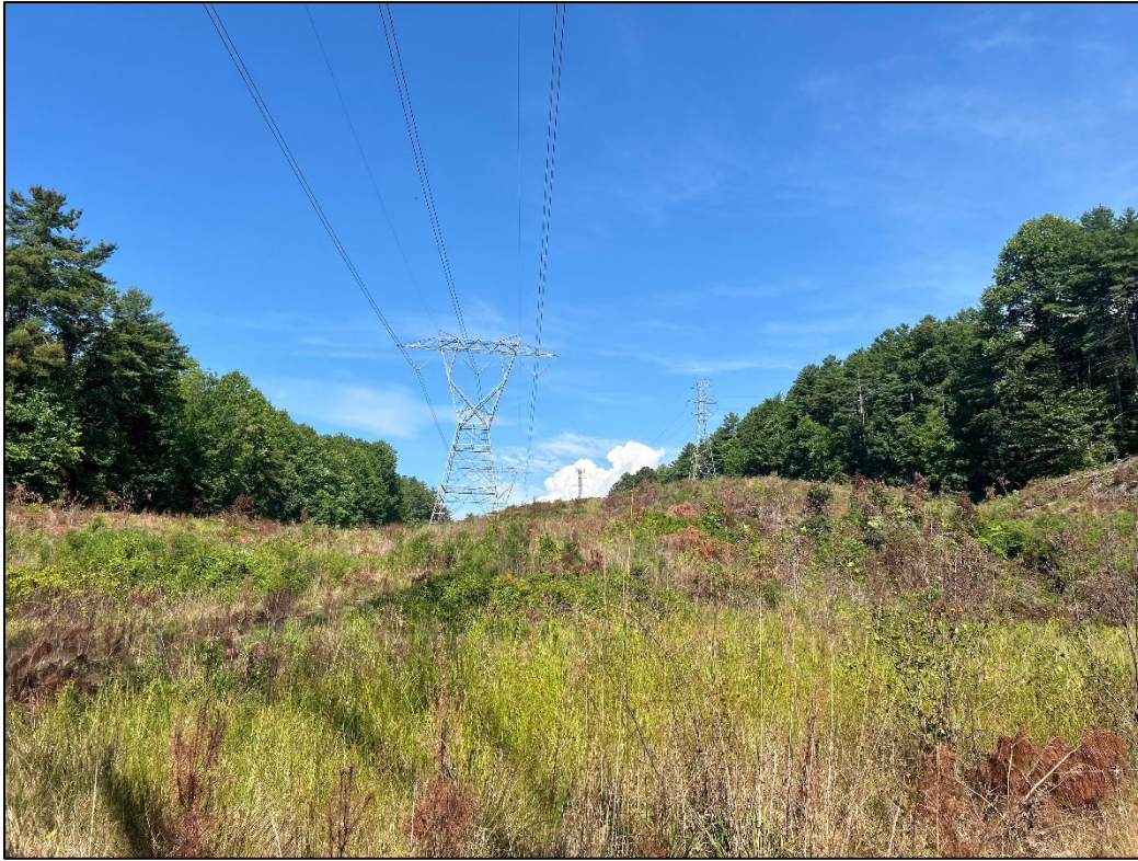
Figure 2-7. Project Primary Transmission Line Corridor Maintained Using Integrated Vegetation Management (As Viewed from the Transmission Line Corridor)
