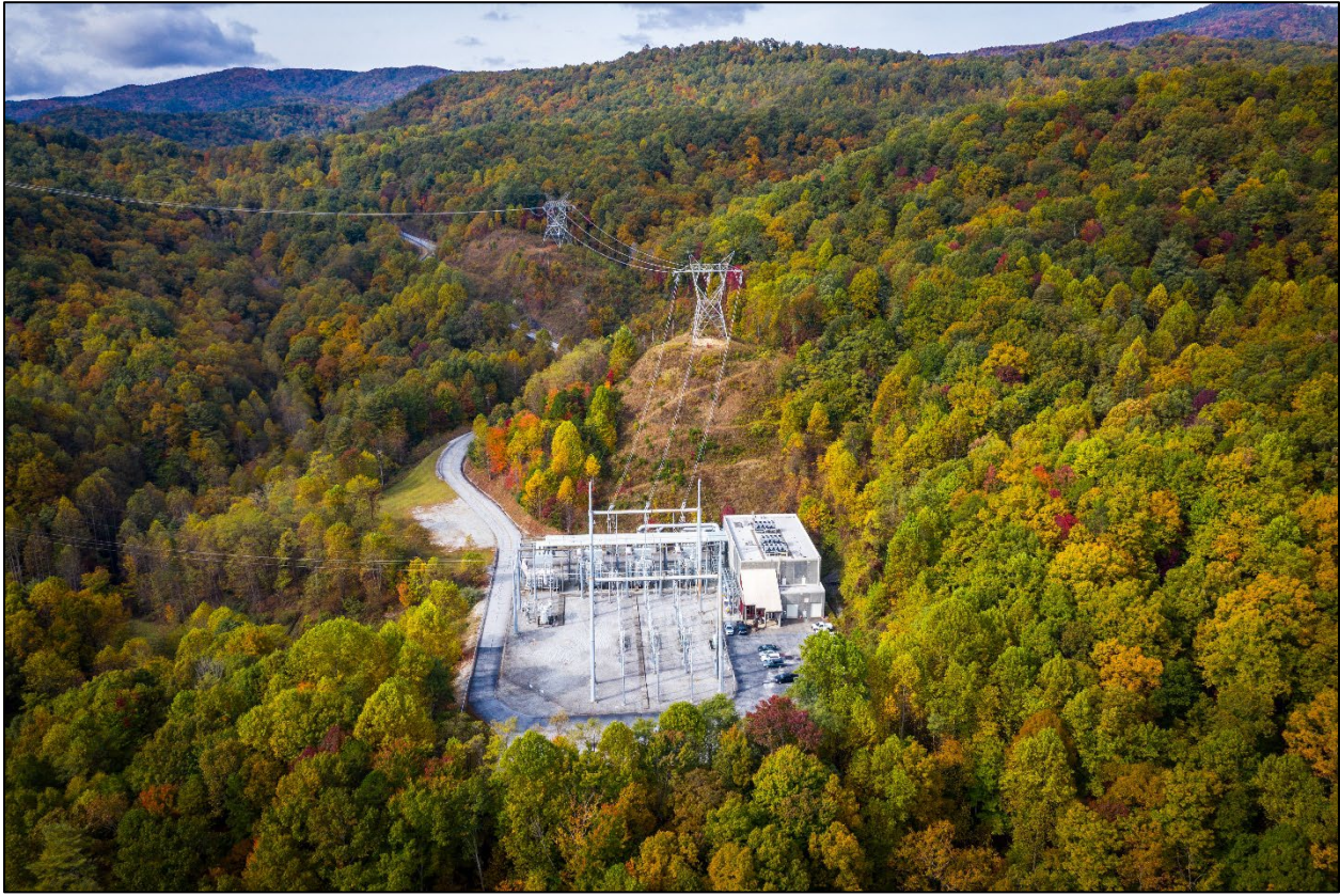
Figure 2-5. Aerial View of the Equipment Building, Transformer Yard, and Switchyard
