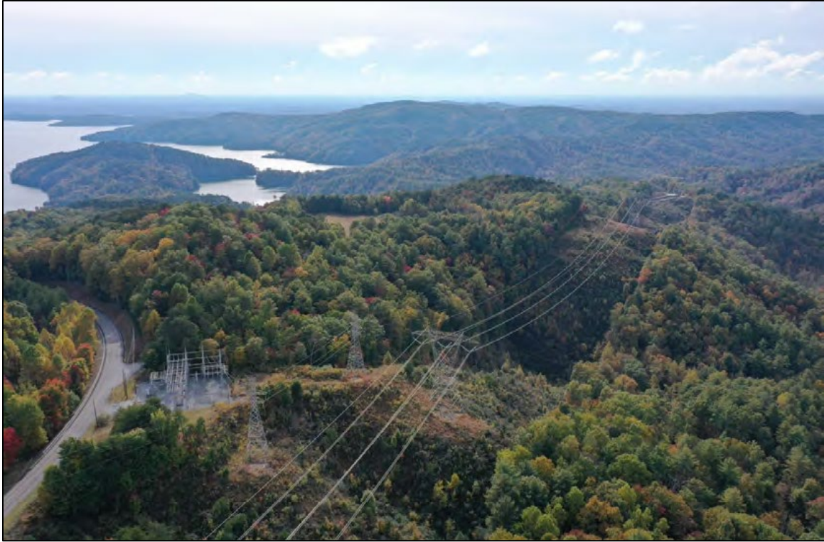
Figure 2-6. Aerial View of Bad Creek Primary Transmission Line and Corridor Spanning a Ravine
