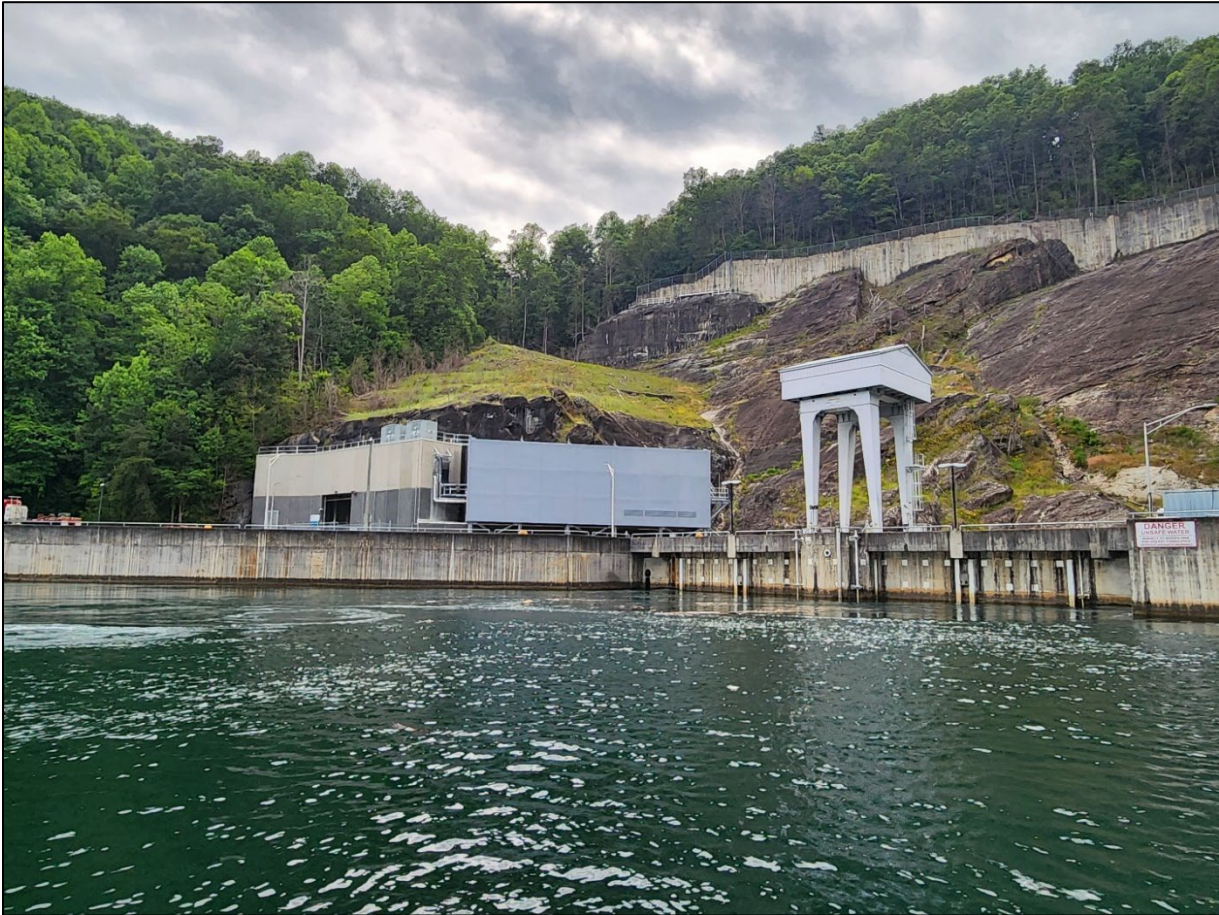
Figure 2-4. Lower Inlet/Outlet Structure and Powerhouse Portal in Whitewater River Cove (As Viewed from Boat Within the Whitewater River Cove of Lake Jocassee)
