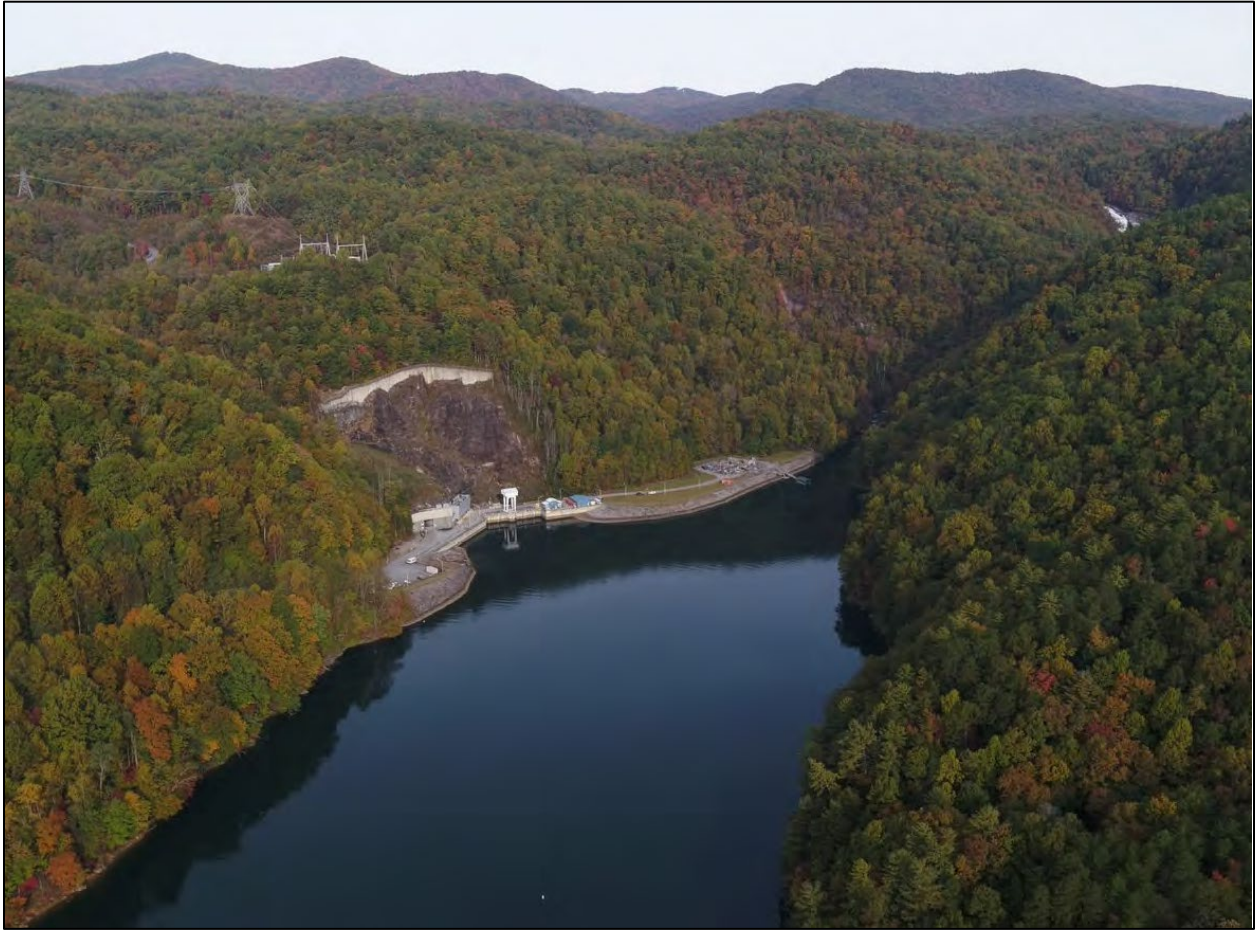
Figure 2-3. Aerial View of the Whitewater River Cove of Lake Jocassee
