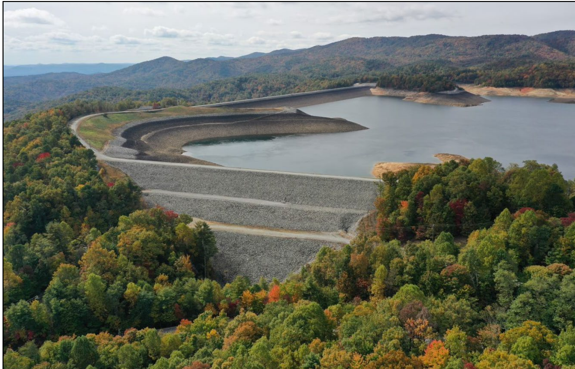
Figure A-3. Aerial View of the Bad Creek Upper Reservoir
