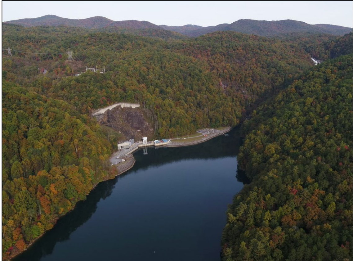
Figure A-4. Lower Reservoir (Whitewater River Arm of Lake Jocassee), Lower Inlet/Outlet Structure, and Powerhouse Portal Area
