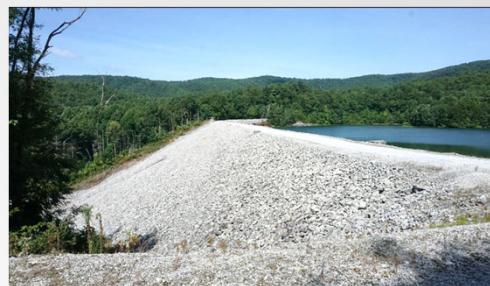
Bad Creek Pumped Storage Project ISR Meeting | 153
