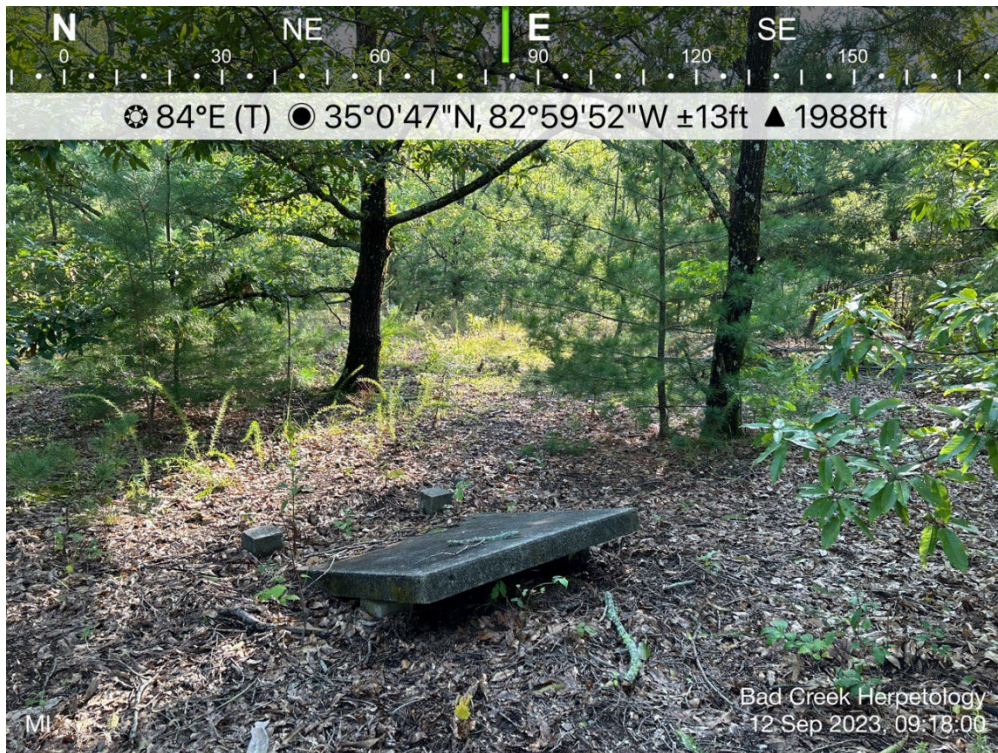
Photograph 16 – Area F, structure
